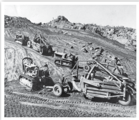
Seabees with 62nd Naval Construction Battalion working around the clock to build an airstrip and camp areas on Iwo Jima.
