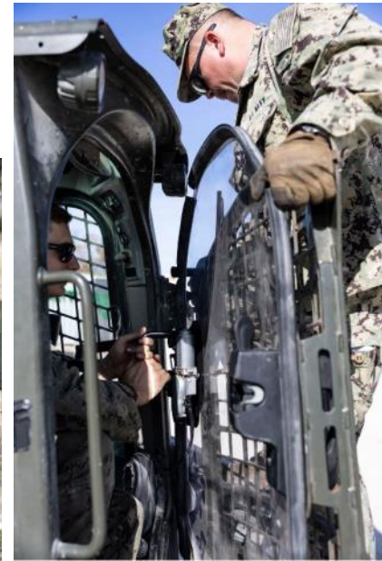
Construction Mechanic 2nd Class Jonathan MarreroGuerra, right, and Construction Mechanic Constructionman Brian Richmond, install a door on a skidsteer on Camp Mitchell in Rota, Spain
