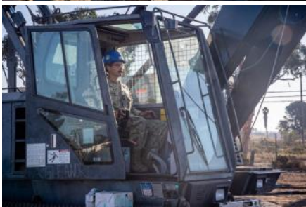
Equipment Operator 3rd Class Joseph DeJohn operates a crane during a field training exercise (FTX) onboard Naval Base Port Hueneme
