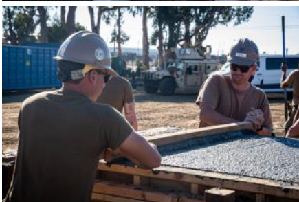
Seabees assigned to Naval Mobile Construction Battalion (NMCB) 5 place concrete during a field training exercise (FTX) onboard Naval Base Port Hueneme
