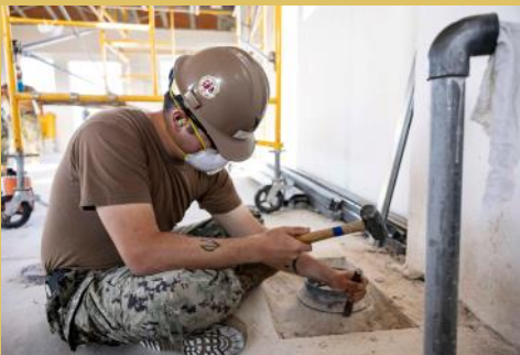
Seabees are continuing their hard work on the military working dog project in Rota, Spain. They are leveling floor drainage, installing electrical outlets, and installing a new silt fence around the site.
