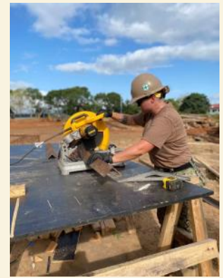
Top Left: Builder 2nd Class David Derosset checks soil compaction prior to concrete placement for a tension fabric structure to be used as a maritime training facility. Top Right: Steelworker 1st Class Brittany Harkovich cuts angle irons for concrete placement. Lower L-R: 1. Marines, assigned to the 8th Engineering Support Battalion (8th ESB), and Seabees, assigned to NMCB 133, cut concrete forms. 2. Seabees and Marines mix concrete. 3. Senior Chief Constructionman Jason Fletcher directs the mixing of concrete and aggregate. 4 & 5. Seabees and Marines place concrete.
