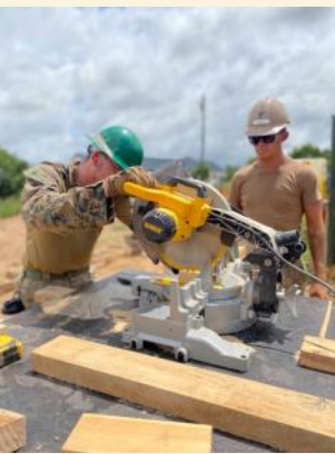
Top Left: Builder 2nd Class David Derosset checks soil compaction prior to concrete placement for a tension fabric structure to be used as a maritime training facility. Top Right: Steelworker 1st Class Brittany Harkovich cuts angle irons for concrete placement. Lower L-R: 1. Marines, assigned to the 8th Engineering Support Battalion (8th ESB), and Seabees, assigned to NMCB 133, cut concrete forms. 2. Seabees and Marines mix concrete. 3. Senior Chief Constructionman Jason Fletcher directs the mixing of concrete and aggregate. 4 & 5. Seabees and Marines place concrete.
