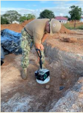
Top Left: Builder 2nd Class David Derosset checks soil compaction prior to concrete placement for a tension fabric structure to be used as a maritime training facility. Top Right: Steelworker 1st Class Brittany Harkovich cuts angle irons for concrete placement. Lower L-R: 1. Marines, assigned to the 8th Engineering Support Battalion (8th ESB), and Seabees, assigned to NMCB 133, cut concrete forms. 2. Seabees and Marines mix concrete. 3. Senior Chief Constructionman Jason Fletcher directs the mixing of concrete and aggregate. 4 & 5. Seabees and Marines place concrete.
