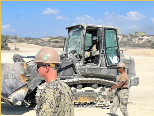
Our Cyprus detail is making progress clearing and leveling at the helicopter landing pad construction site.
