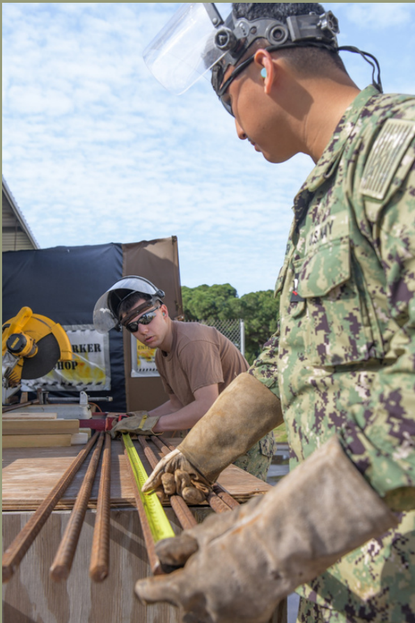
In Camp Mitchell, Naval Station Rota, Spain, LUCKY ELEVEN's Steelworkers have been cutting up rebar to use in structural reinforcement.
